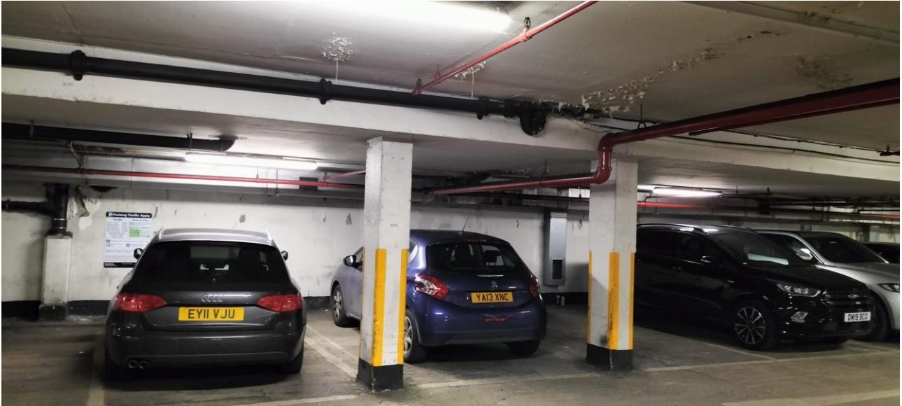
Photograph No. 6 – View within car park.
