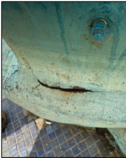
Cracks in existing base (recently patched up and repainted)
