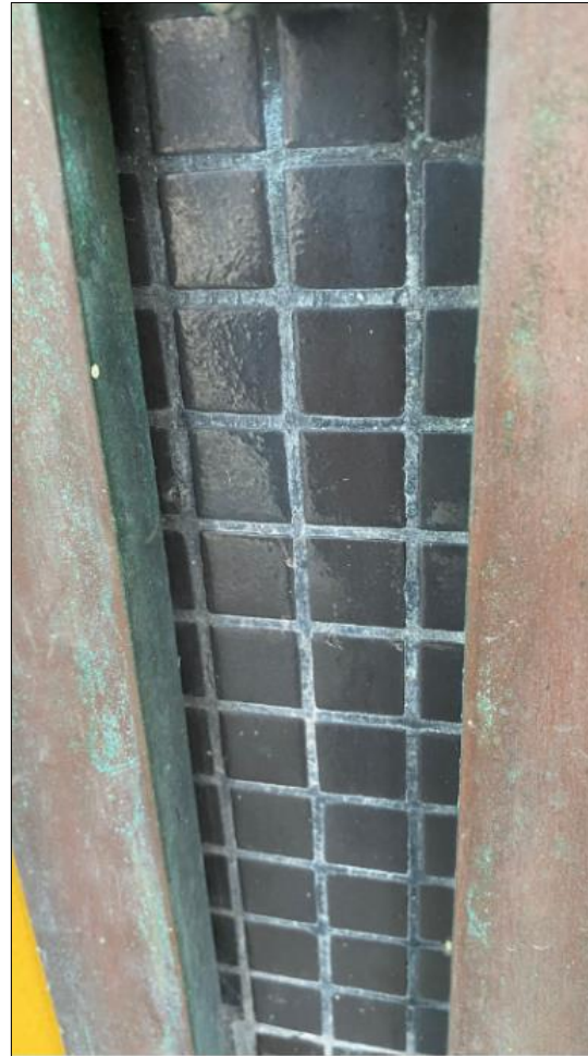
Surviving area of original black ceramic mosaic tiles
