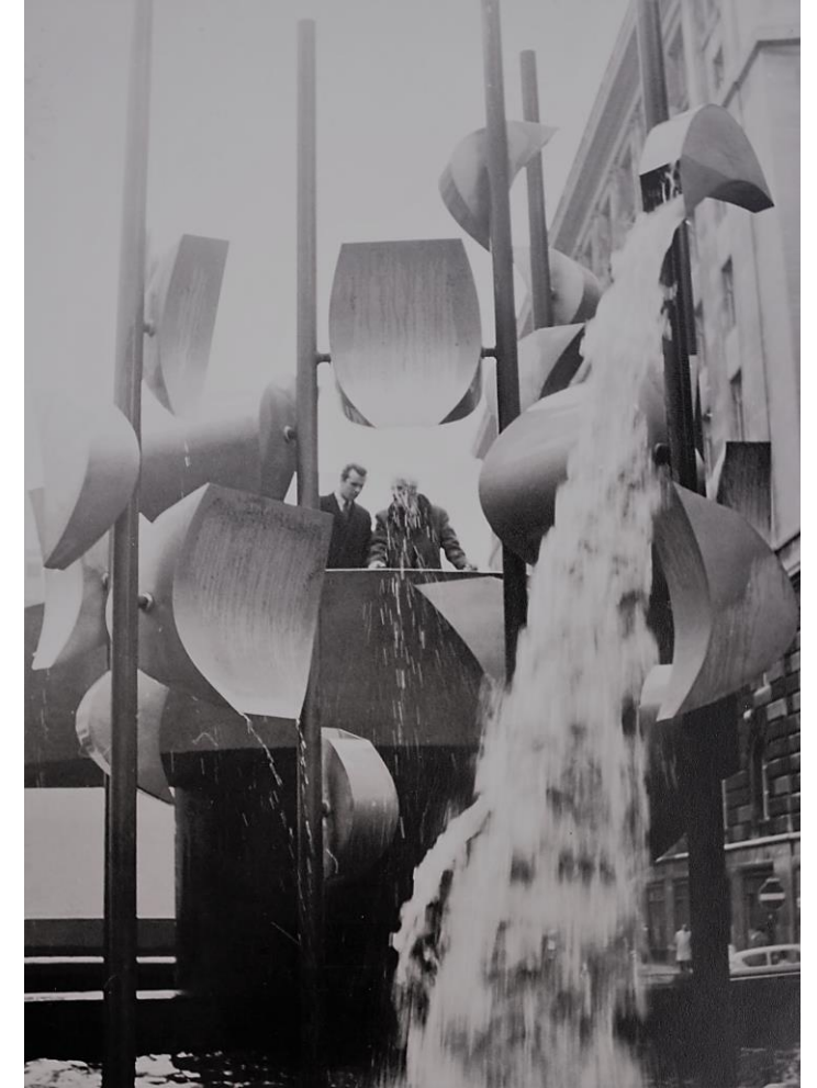
Original tipping frequencies restored but future wear of bearings and leakages prevented
