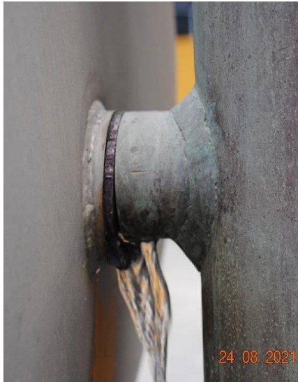
Drop & leak from larger 'bucket' Cause as for smaller buckets
