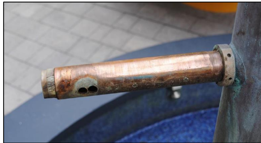
Worn bronze supply pipe/axle causing leaks between axle and 'Tufnol' sleeve
