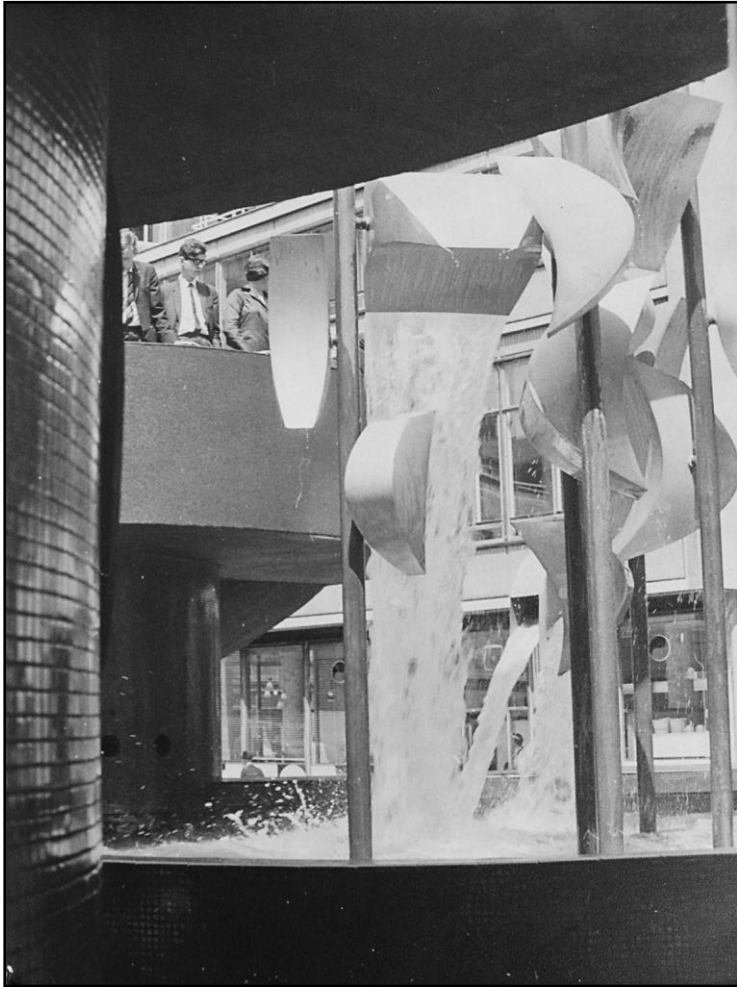
Glossy tiled finish restored with more durable polished Dark Blue Grey Welsh slate mosaic tiling
